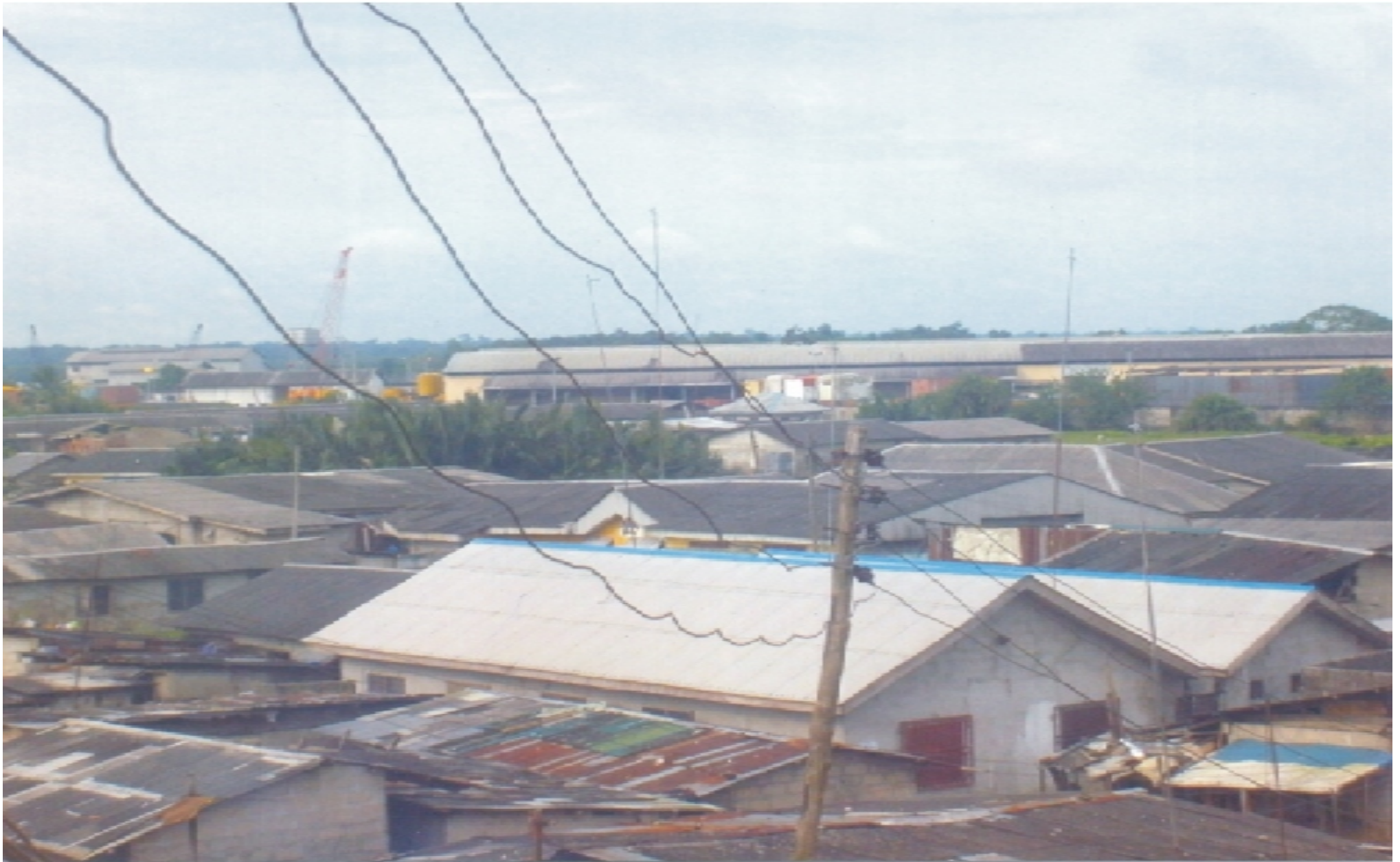
Photograph of a segment of Abonnema Wharf/Njemanze waterfronts marked for demolition
